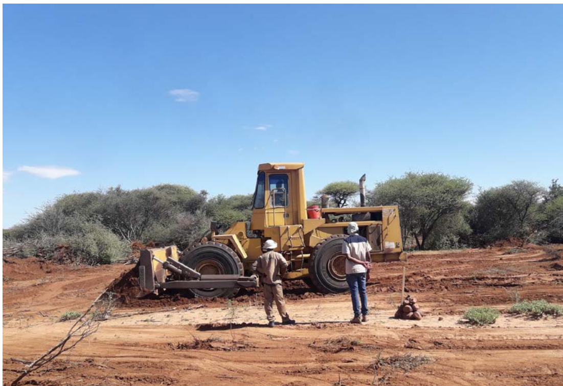
Figure 1: Site clearance at Joubira in preparation for drilling.
