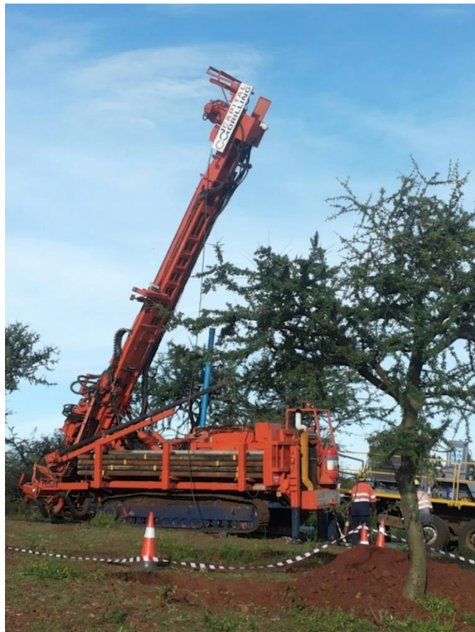
Track Mounted Multi-purpose RC/Diamond Rig at Winston
